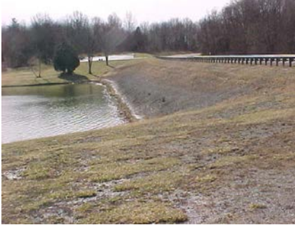
View of upstream slope from right abutment
