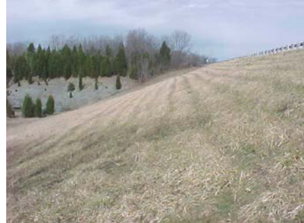
Downstream slope viewed from left abutment
