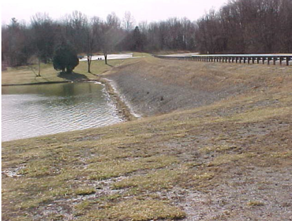
View of upstream slope from right abutment
