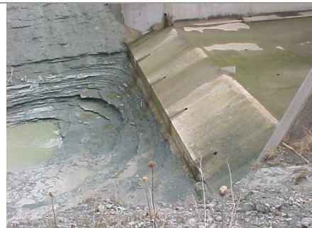
End of chute, 800 feet downstream of control section
