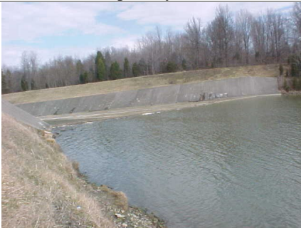
Spillway inlet
