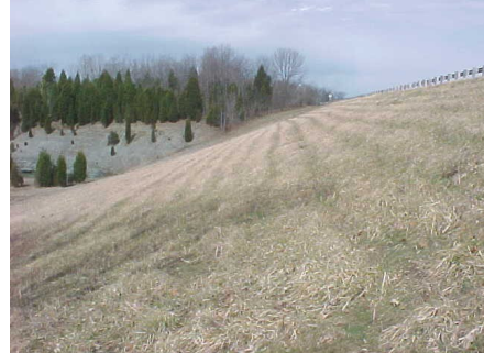
Downstream slope viewed from left abutment
