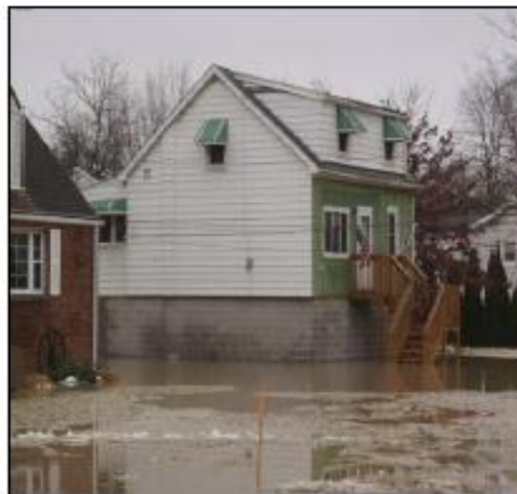
Murray Road - Elevated structure during the February 28, 2011 flood event.
