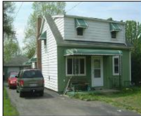
Murray Road Property – Before Elevation
