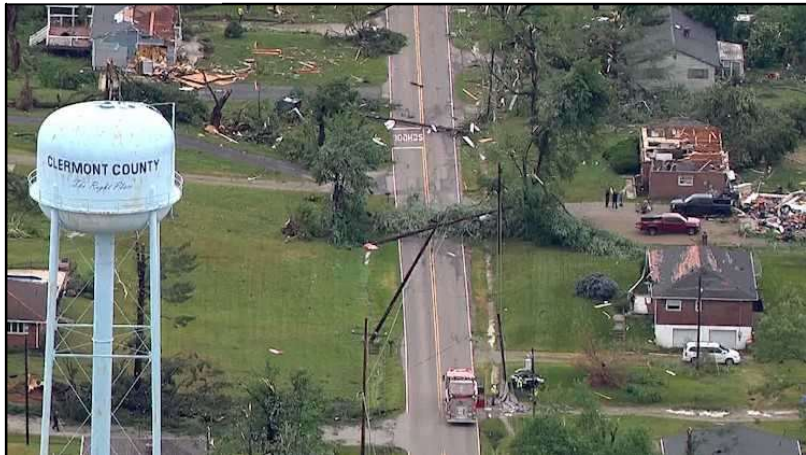
Tornado Damage – Goshen Township
