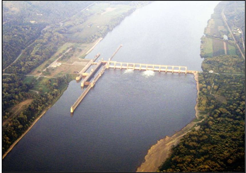
Captain Anthony Meldahl Locks & Dam located between Neville and Chilo
