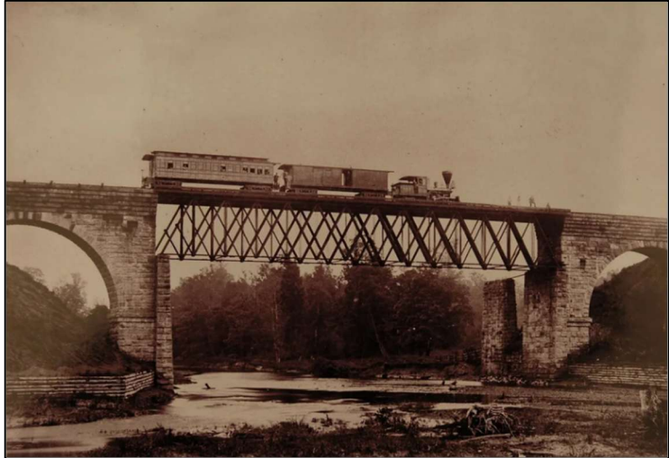
Railroad Bridge that collapsed, 1879
