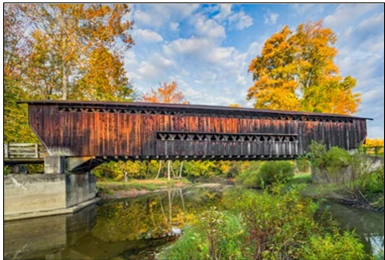
Historic Benetka Road Covered Bridge
