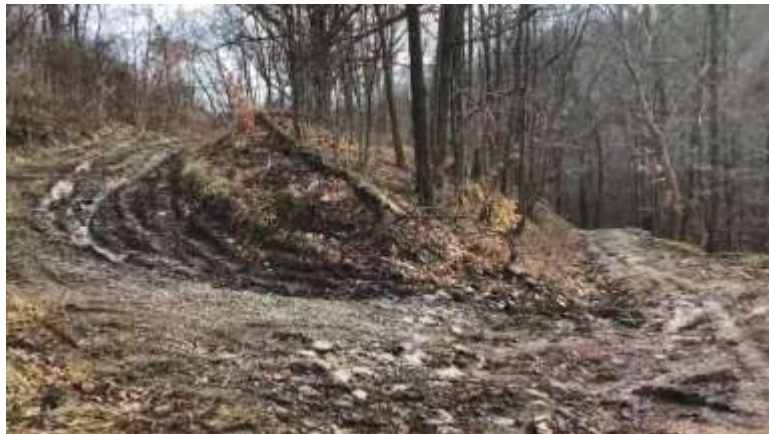
FIGURE 5 LANDSLIDE IN BELMONT COUNTY, 2018
